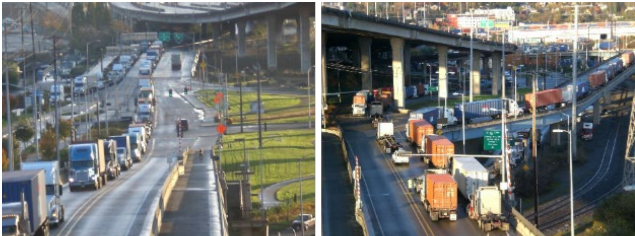
Figure 1: Truck Queuing on SW Spokane Street and Bridge Across the Duwamish River
